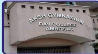
Multipurpose Gymnasium Hall
